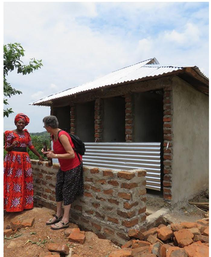
Roofing is generally corrugated metal. A ceiling is added where possible to provide insulation and reduce heat build up in the middle of the day.
